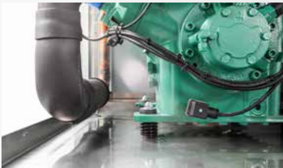
Anti-vibration springs
