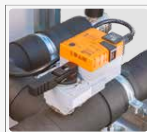
Power control via three-way valve
