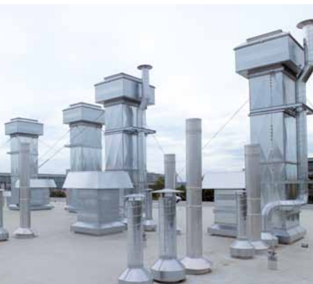
Exhaust Air Ducts with Deflectors
