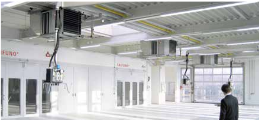
WD-A supply air unit - heating medium: hot water
