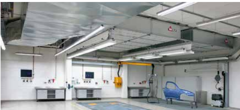
Air supply via filter ceiling
