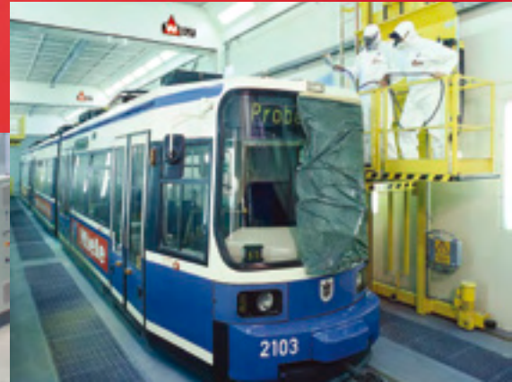
Large-space Spray Booths for Rail Vehicles Site: SWM Munich
