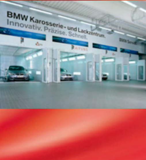
Spraying and Drying Booth TAIFUNO® Site: BMW Munich-Garching
